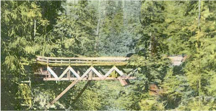
The wooden footbridge, date unknown. Its triangular "Howe Truss" design made it especially strong. NVMA 2720
